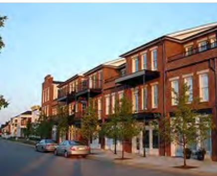
Larger buildings should utilize design techniques that reduce their apparent height and width
