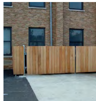
Service features such as garbage containers should be shielded from view in an enclosure compatible with the building architecture
