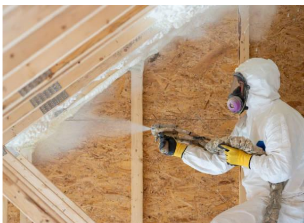
Spray Foam Insulation
