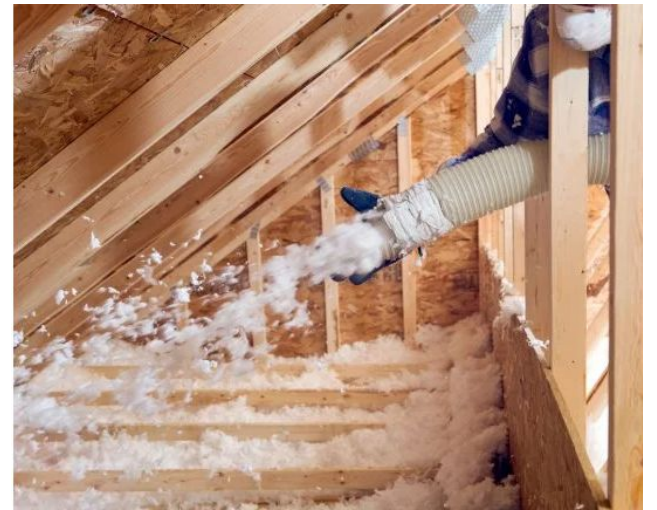
Blown-In Insulation Courtesy to North Tarrant Heat & Air
