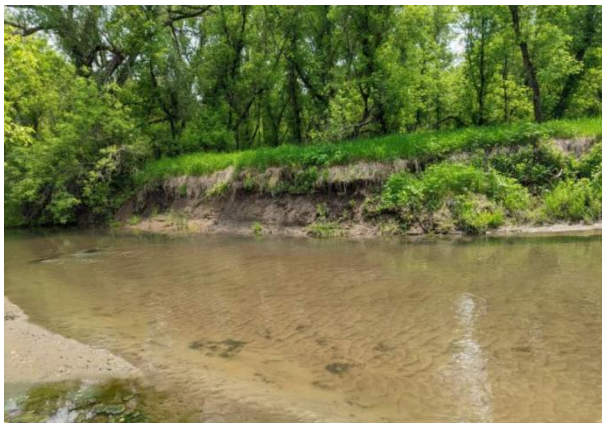
Bank erosion along Pine Creek.
